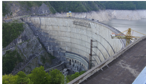
The 227 meters high arch dam of the Enguri Dam in Georgia.
