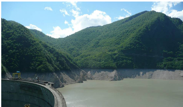
Compared with other dams, Enguri Lake has a very high annual water level fluctuation of around 100 meters.
