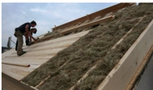
Roof insulation with bast fibres.
